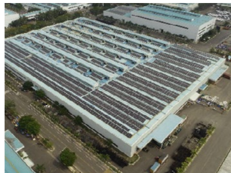
A photovoltaic power generation facility in HMI
