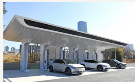
E-pit charging station
